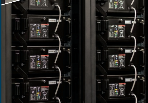
BATTERIES IN AN ADVANCION NODE
