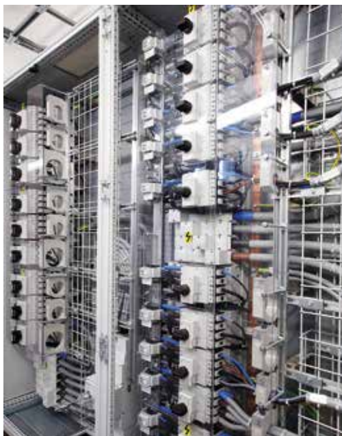
The power distribution system of the production plant: Eaton's 160 A - 630 A NZM compact circuit breakers are used
