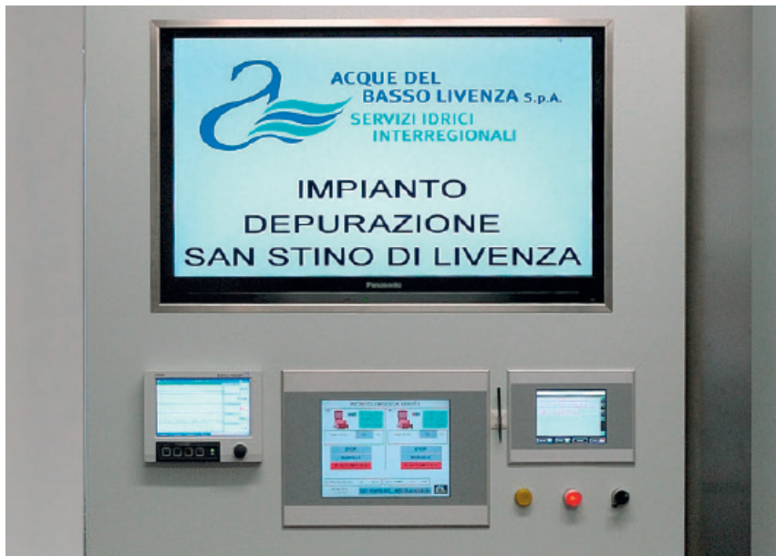
The plant is being controlled and operated via an industrial PC and two touch display control units, the integrated remote control functionality helps increase availability.
