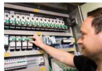
Thanks to the SmartWire-DT intelligent connection and communication system the wiring is reduced by approximately 40%
