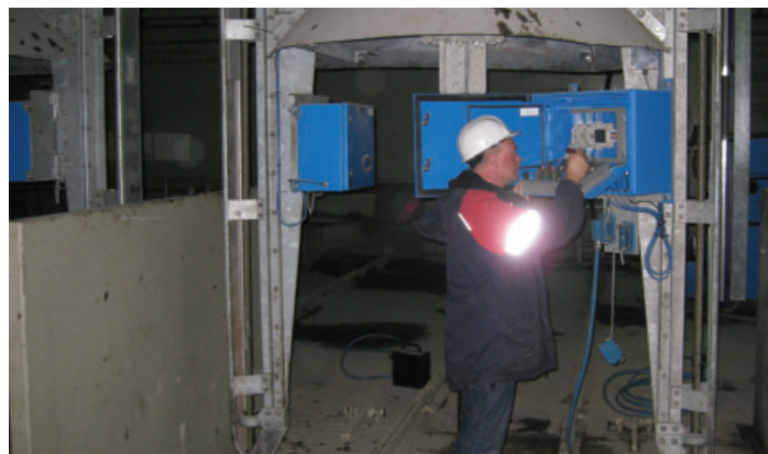
Mounting the main cubicle for wireless communication
