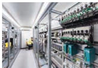
The control station and the electronic technology were shipped in one container so that the crushing operation modernization project could be completed as quickly and smoothly as possible.
