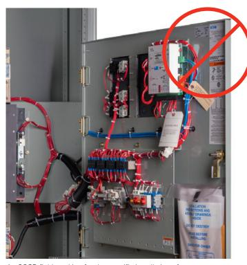
An SCCR field marking for the specific installation of emergency system transfer equipment must be made on the enclosure exterior – not the interior. The manufacturer's nameplate SCCR marking is on the inside
